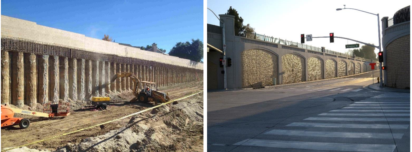
Figure 6. Secant Pile Wall Construction In-Progress and Completed
