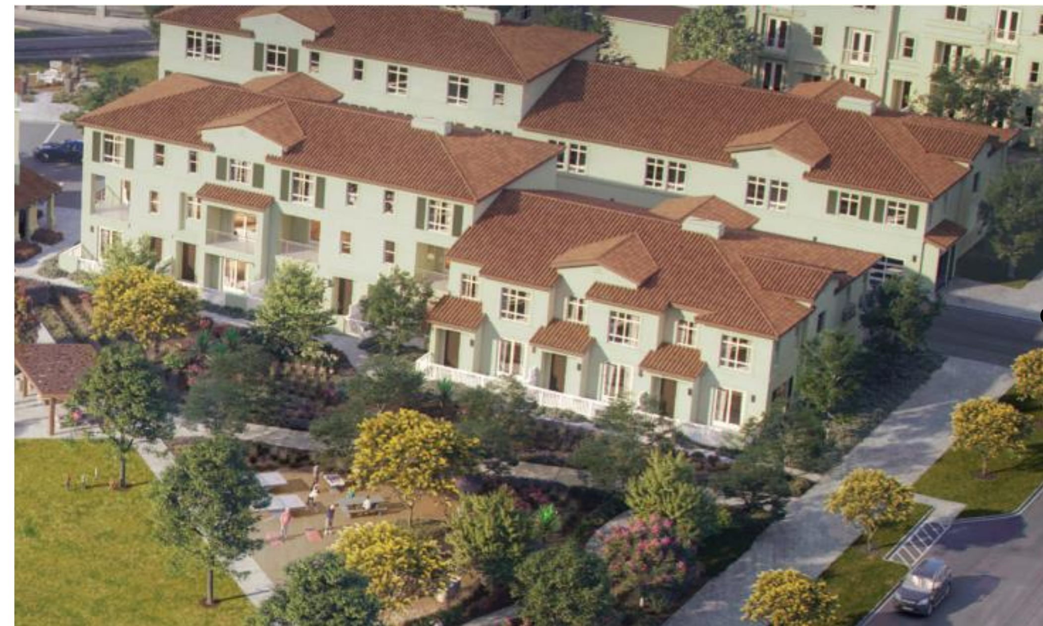
2- AND 3-STORY TOWNHOMES 123 units
