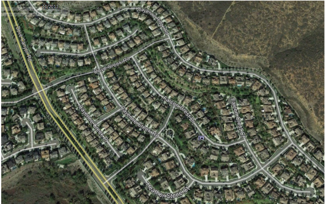
Figure 4. Example higher density development. Homes are ignition resistant and excludes readily ignitable vegetative fuels throughout and provides a perimeter fuel modification zone. This type of new development requires fewer fire resources to defend and can minimize the likelihood of on-site fires spreading off-site.
