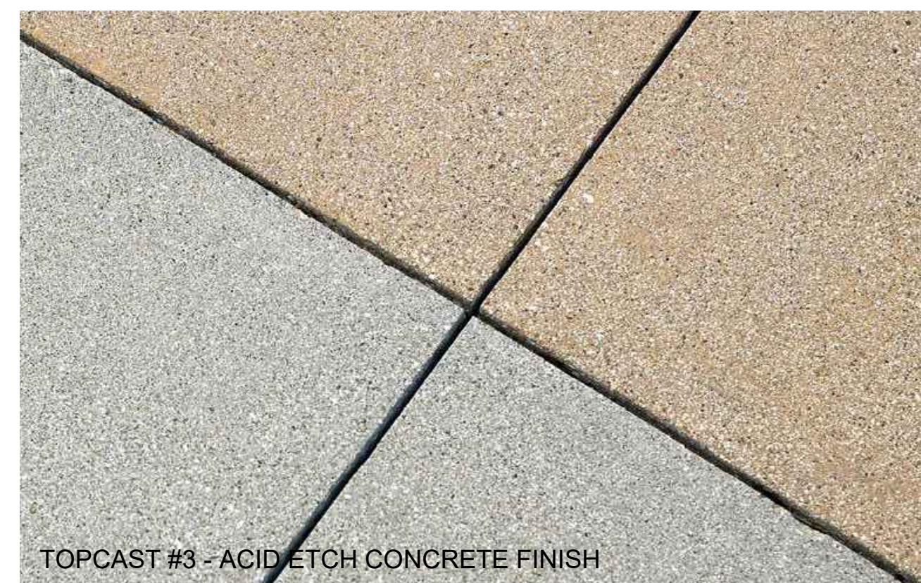
TOPCAST #3 - ACID ETCH CONCRETE FINISH
