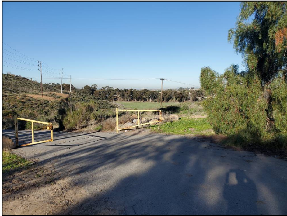
View of access road adjacent to southeast corner of the Subject Property.
