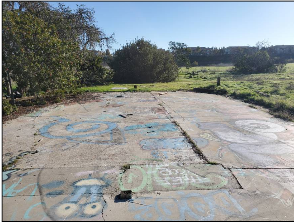
View of former building pads.
