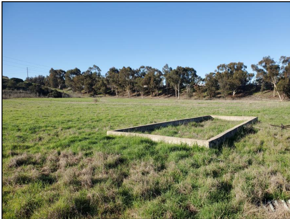
View of former building pads.
