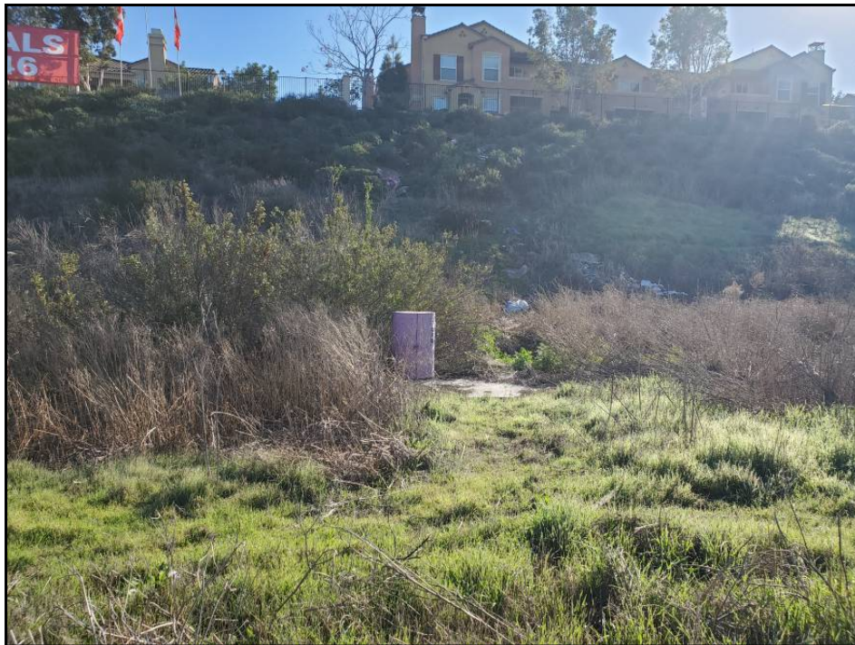
View of Otay Mesa Water District infrastructure along eastern boundary of the Subject Property.
