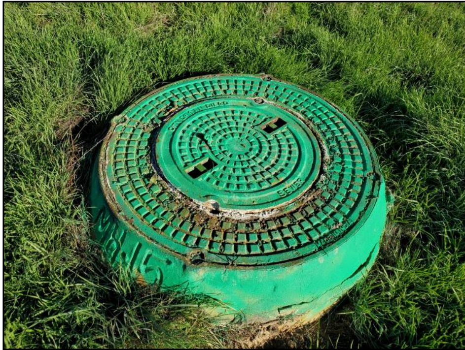
View of manhole cover.
