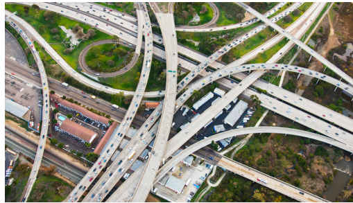
Interchange Where a freeway and a major road or other freeway cross each other.
