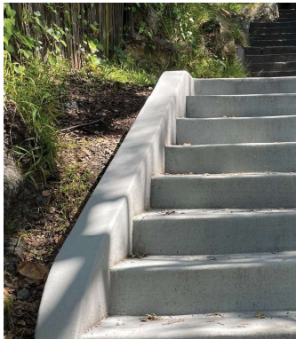
Concrete Cheek Wall at Stairs
