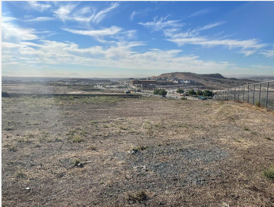
Photograph 17: Photograph looking south along the western property boundary of the Otay Ranch Village 7 South Project site. Photograph taken standing above La Media Road, near the existing entrance into the project site. Note the existing construction taking further south of the project site.
