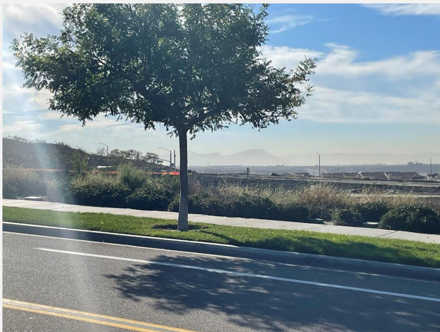
Photograph 18: Photograph looking south towards construction currently taking place south of the Project site. Photograph taken standing along Santa Luna Street, near the intersection of Santa Luna St. and Magdalena Ave.
