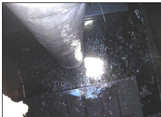
Removal of trash, sediment and debris.
