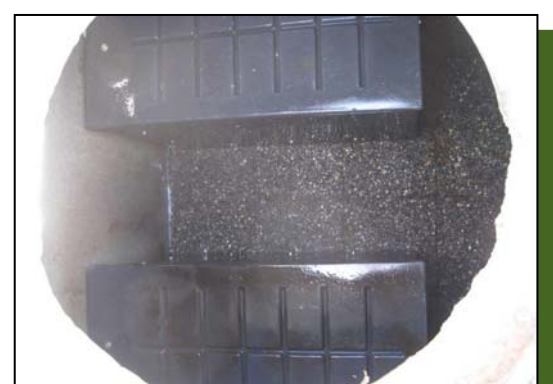
Fully cleaned separation chamber.
