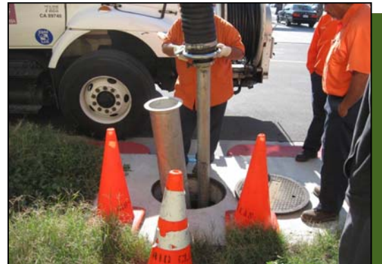
Insertion of vacuum hose into separation chamber.
