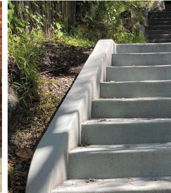
Concrete Cheek Wall at Stairs
